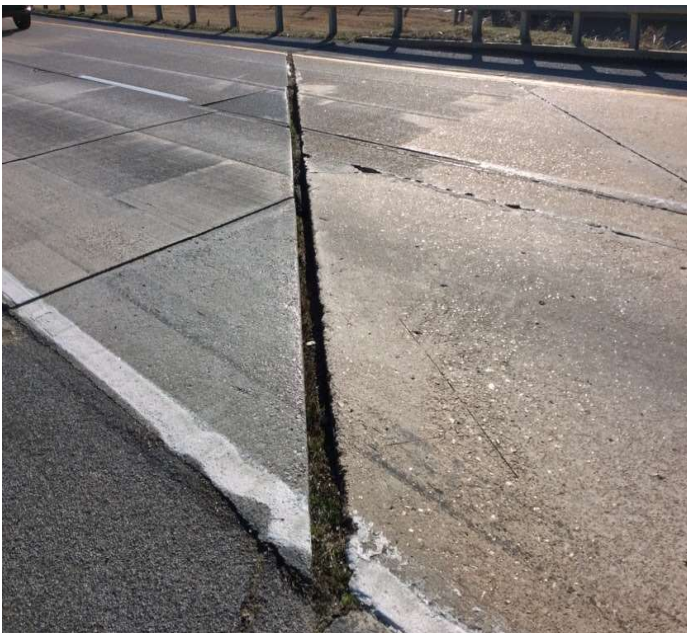
PHOTO 1 Description Gap between approach slab and approach roadway
