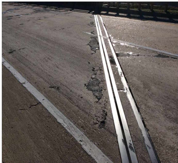
PHOTO 1 Description Spalls along joint over bent 1
